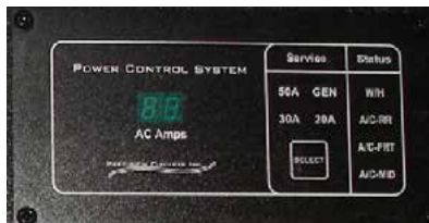
50A System Panel
