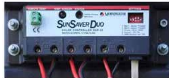
Solar Panel Control (location may vary by model)
